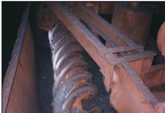
Old screw showing weld overlay repairs
